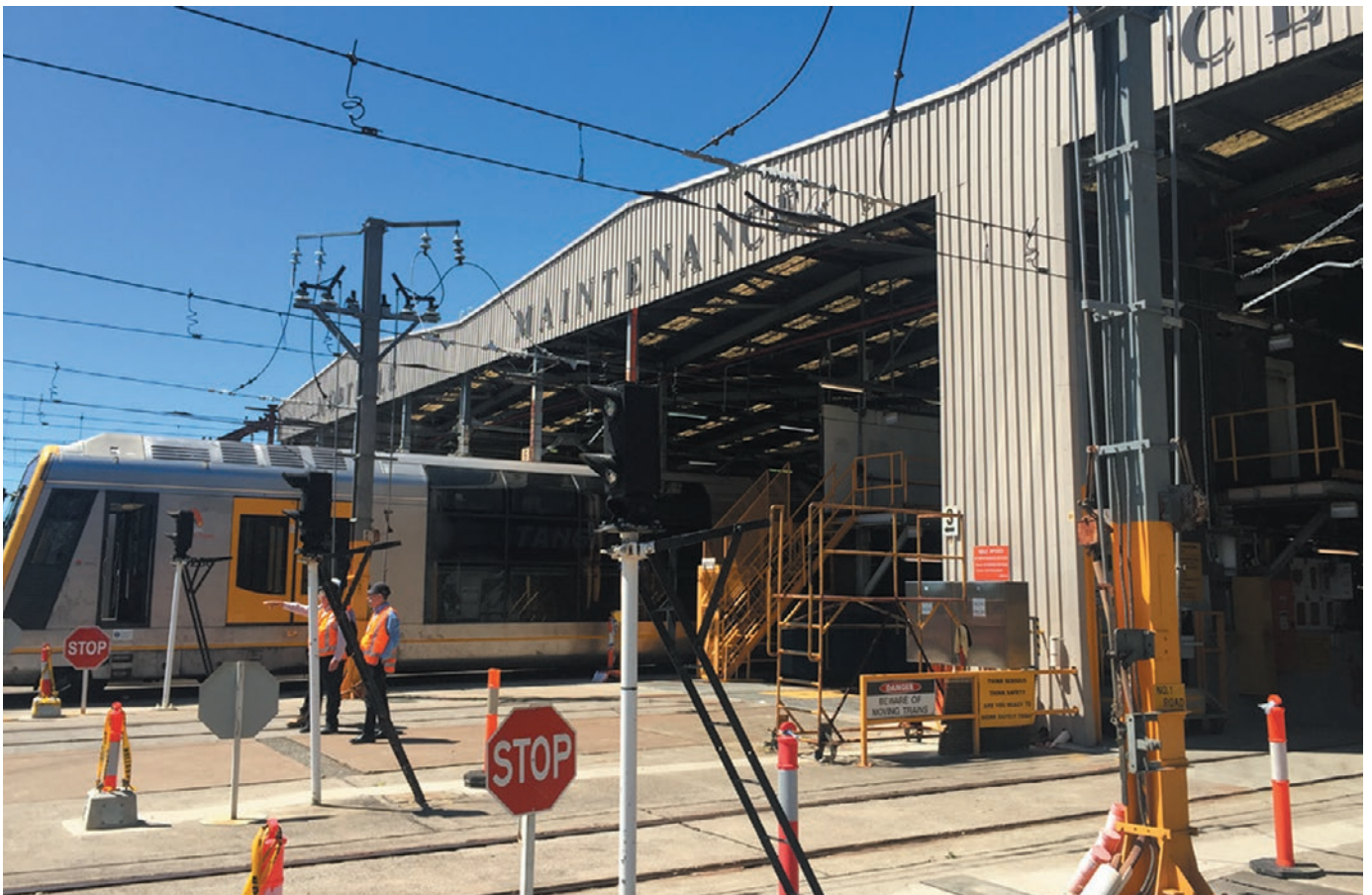
The existing Mortdale Maintenance Centre.
