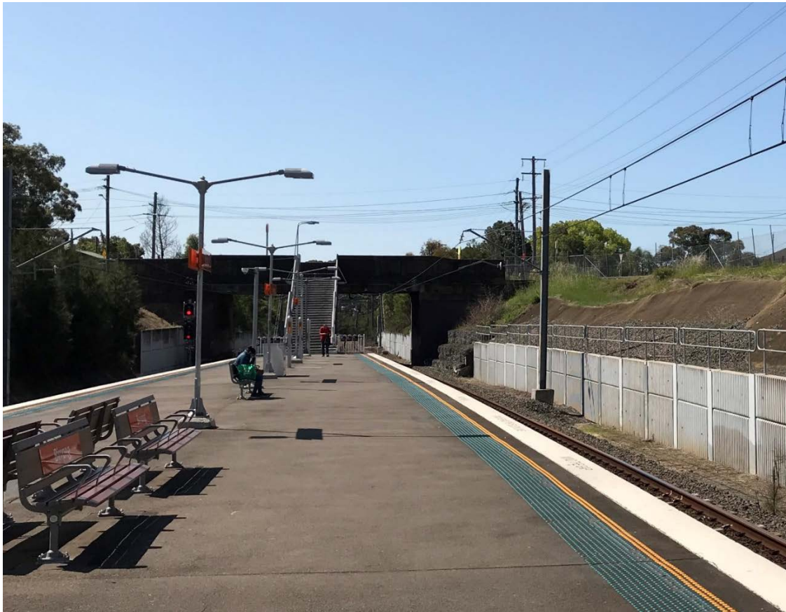
Figure 5 View north along platform 1 towards the existing stairs and footpath/road overbridge.
