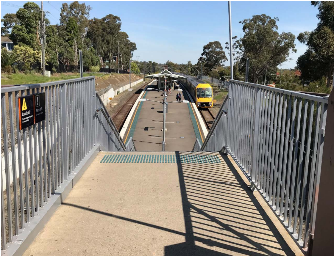
Figure 6 View south to the station from the footpath on Avalon Street overbridge.
