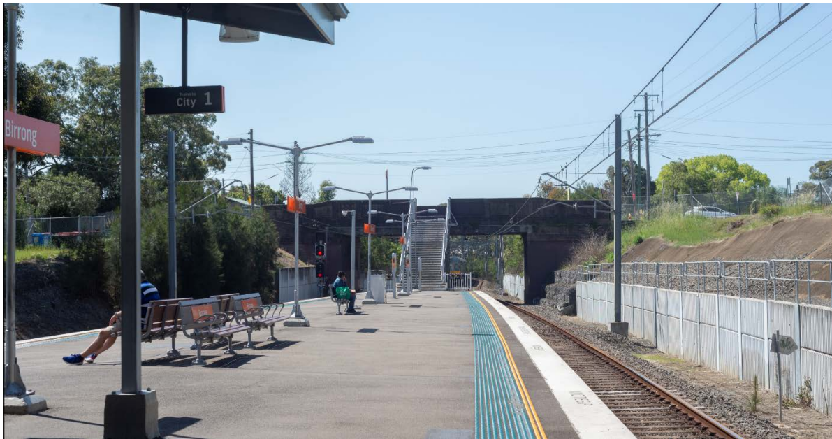
Figure 11 Viewpoint 1 – existing view from eastern side of station building
