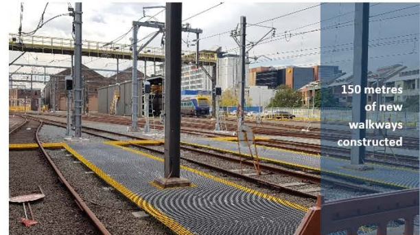
Five train buffer stops replaced
