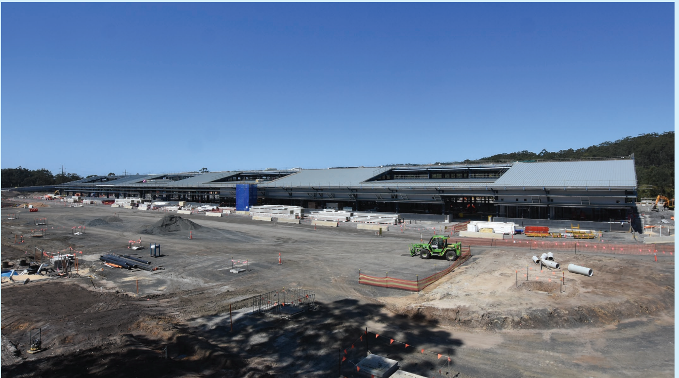
View of the Maintenance Facility building facing the rail corridor.
