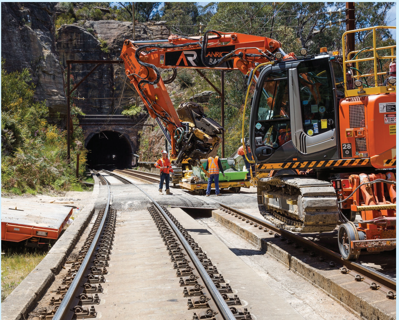
Trackwork between Tunnel 8 and 9, Ten Tunnels Deviation
