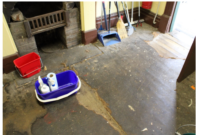
Figure 5.58: Original timber floorboards within storage room (Source: Jacobs 2020)
