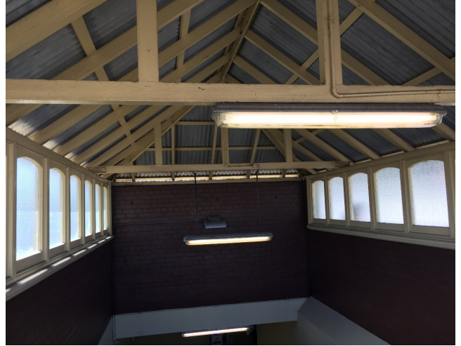
Figure 5.33: Detail of roof covering over stairwell, facing north (Source: Jacobs 2020)
