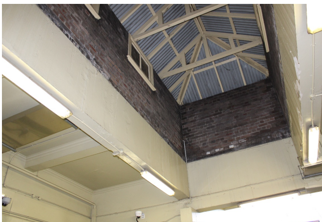
Figure 5.28: Northern lantern vaulted roof viewed from subway (Source: Jacobs 2020)
