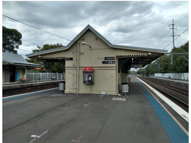
Figure 5.53: Platform 2/3 building, facing south (Source: Jacobs 2020)
