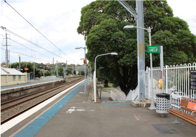
Figure 5.47: Entrance to Platform 4, facing north (Source: Jacobs 2020)
