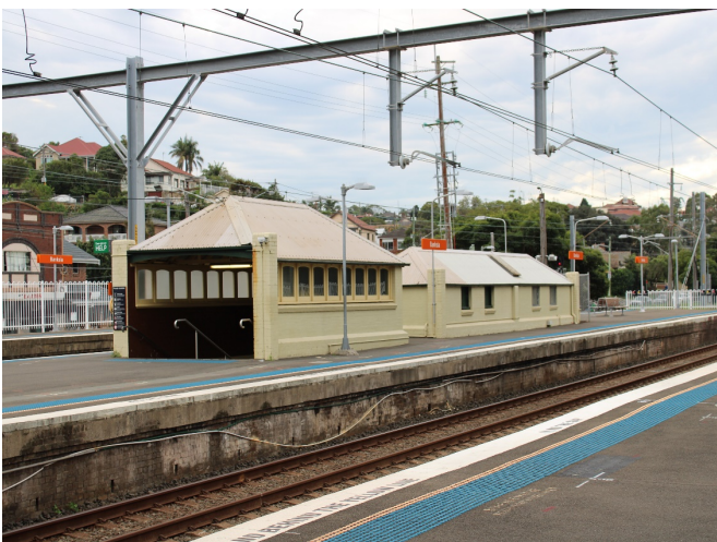
Figure 5.38: Exterior of both lantern structures, facing north west – taken from Platform 4 (Source: Jacobs 2020)
