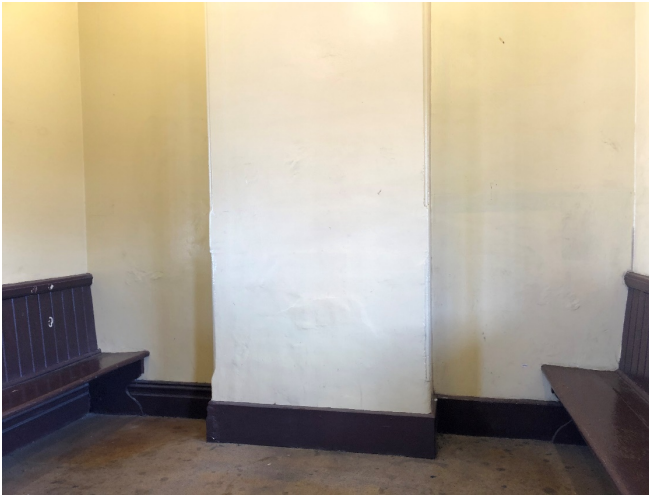
Figure 5.65: Southern interior wall of waiting room (Source: Jacobs 2020)
