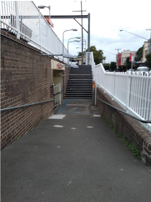
Figure 5.5: Entrance to subway on Railway Street, facing south (Source: Jacobs 2020)
