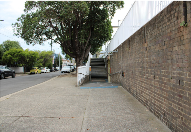
Figure 5.15: Entrance to subway on Hattersley Street, facing south (Source: Jacobs 2020)
