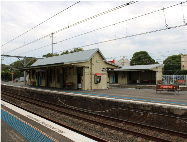
Figure 5.52: View of Platform 2/3 building from Platform 4, facing south west (Source: Jacobs 2020)
