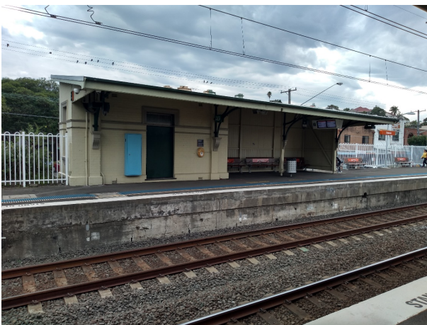
Figure 5.49: View of Platform 1 building from Platform 2, facing west (Source: Jacobs 2020)
