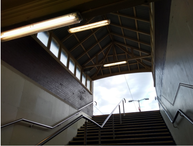
Figure 5.32: Stairwell and roof leading to Platform 2/3, facing south (Source: Jacobs 2020)
