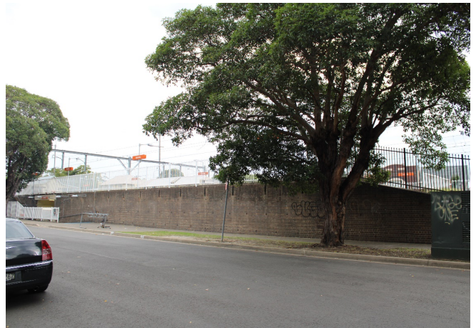
Figure 5.83: Brick retaining wall on Hattersley Street, facing west (Source: Jacobs 2020)
