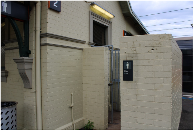
Figure 5.75: Entrance to men's toilet stalls (Source: Jacobs 2020)
