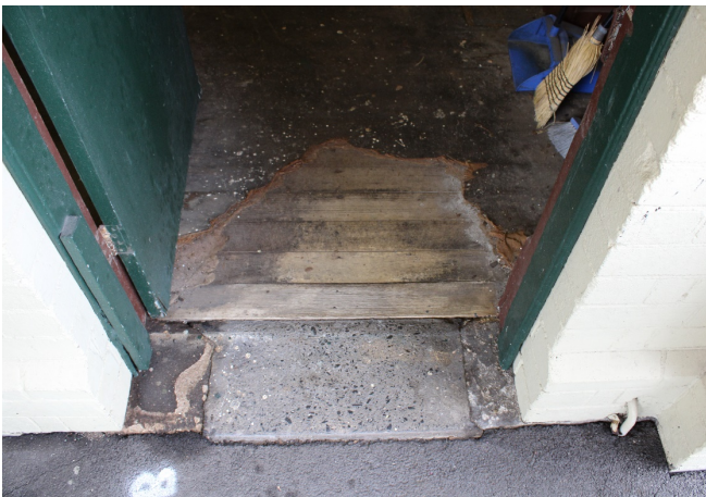
Figure 5.57: Original timber floorboards to storage room (Source: Jacobs 2020)
