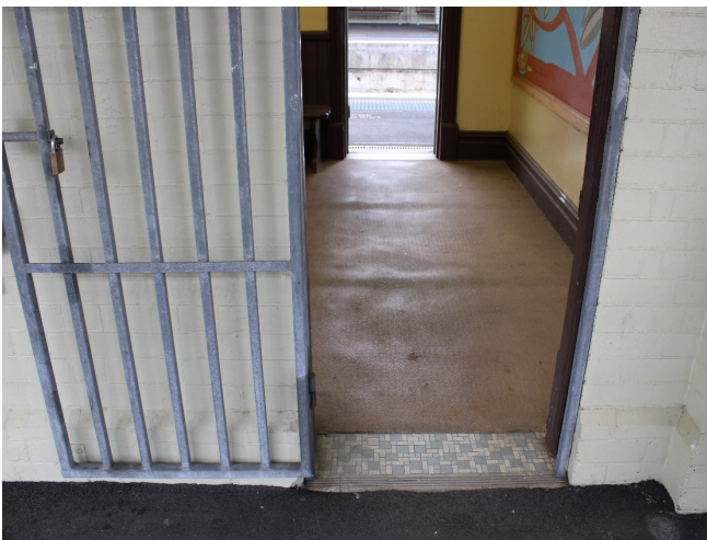
Figure 5.63: Entrance to waiting room, facing west (Source: Jacobs 2020)
