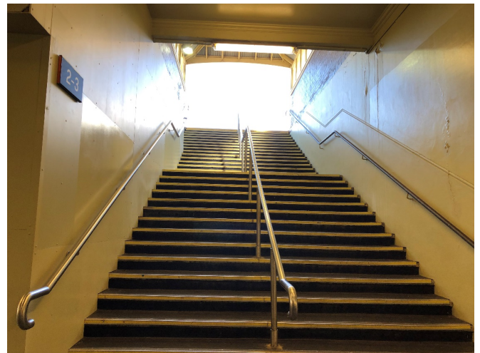
Figure 5.12: Stairs leading from subway to Platform 2/3, facing south (Source: Jacobs 2020)
