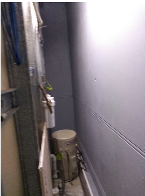
Figure 5.26: Detail on inset and spacing from original interior (Source: Jacobs 2020)
