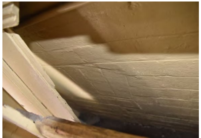
Figure 5.74: View of infilled openings within the cistern room (Source: Artefact Heritage (2020: 37))
