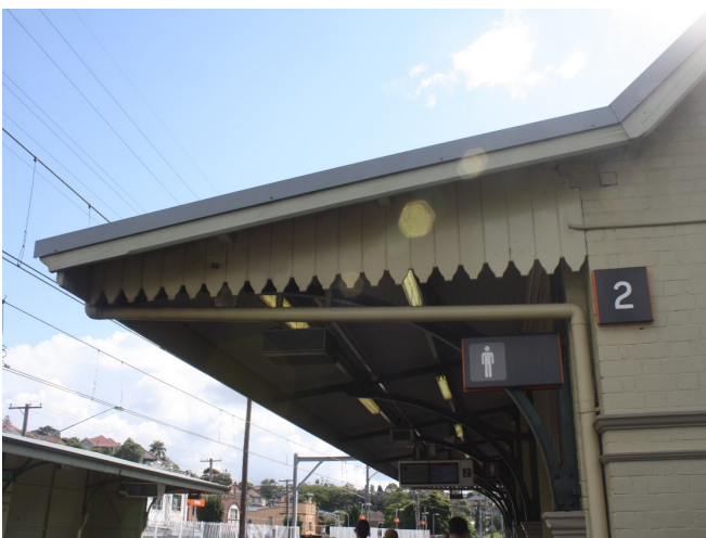
Figure 5.56: Platform 2/3 building roof, facing north (Source: Jacobs 2020)
