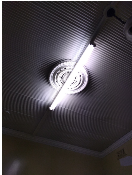
Figure 5.62: Original ceiling and rose within storage room (Source: Jacobs 2020)
