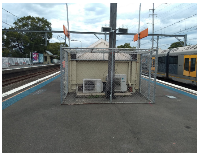
Figure 5.31: Exterior of vaulted roof, located on Platform 2/3, facing south (Source: Jacobs 2020)
