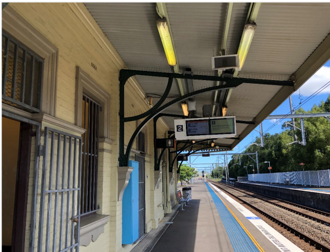
Figure 5.54: Platform 2/3 building, facing south (Source: Jacobs 2020)
