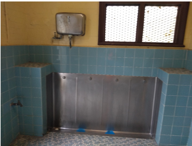
Figure 5.77: Interior of men's toilets (Source: Jacobs 2020)
