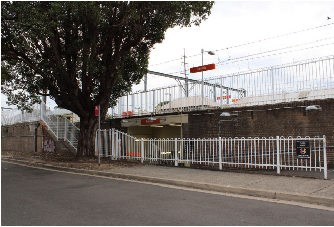
Figure 5.3: Entrance to Banksia Station on Hattersley Street, facing west (Source: Jacobs 2020)
