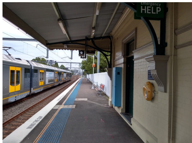
Figure 5.50: Platform 1 building, facing north (Source: Jacobs 2020)
