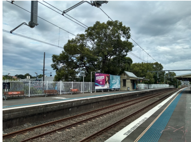
Figure 5.48: View of Platform 4 from Platform 3, facing south east (Source: Jacobs 2020)
