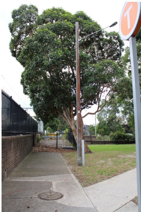
Figure 5.84: Brick retaining wall on Hattersley Street, facing west (Source: Jacobs 2020)
