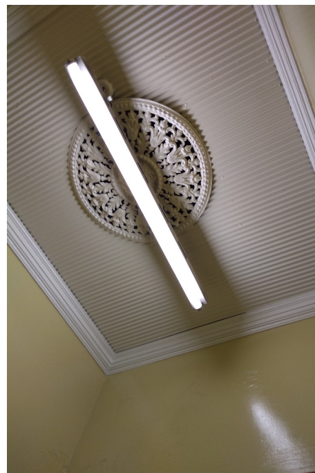
Figure 5.68: Original ceiling and rose within women's waiting room (Source: Jacobs 2020)
