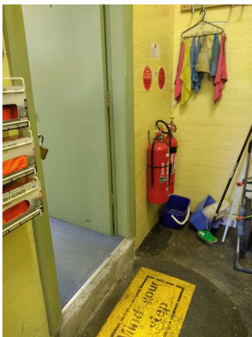
Figure 5.18: Entrance from subway to booking office, facing south west (Source: Jacobs 2020)
