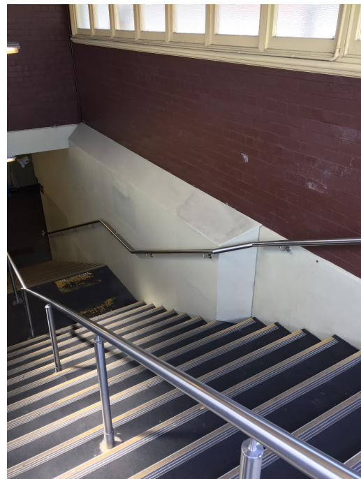
Figure 5.35: Detail of alterations in stairwell, facing north (Source: Jacobs 2020)
