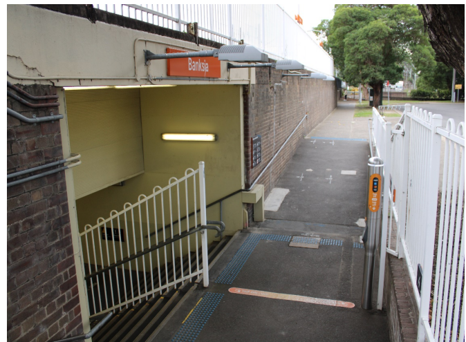
Figure 5.14: Detail of subway entrance on Hattersley Street, facing north (Source: Jacobs 2020)
