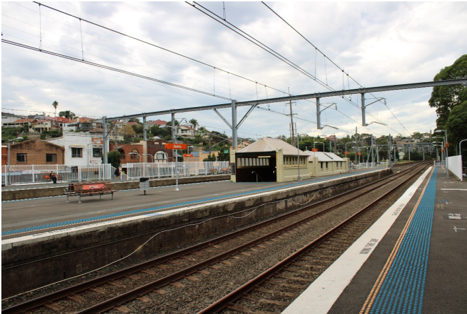
Figure 5.43: View of Platform 3 from Platform 4, facing north west (Source: Jacobs 2020)
