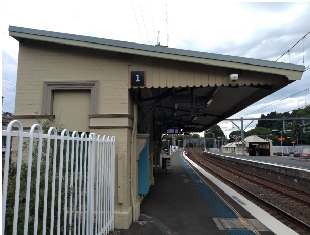
Figure 5.51: Platform 1 building, facing north (Source: Jacobs 2020)
