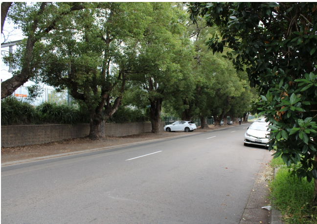
Figure 5.82: Brick retaining wall on Railway Street, facing south (Source: Jacobs 2020)
