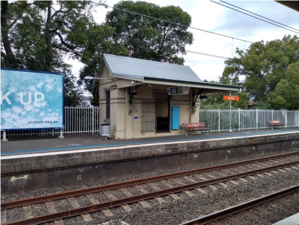
Figure 5.78: View of Platform 4 building from Platform 3, facing south east (Source: Jacobs 2020)
