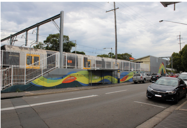
Figure 5.1: Entrance to Banksia Station on Railway Street, facing east (Source: Jacobs 2020)
