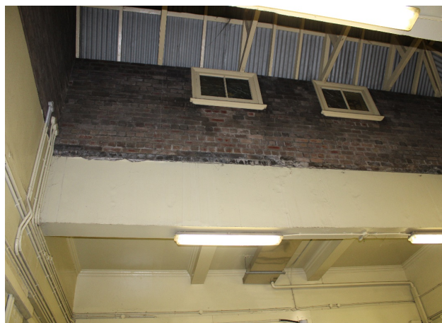
Figure 5.29: Northern lantern vaulted roof viewed from subway (Source: Jacobs 2020)
