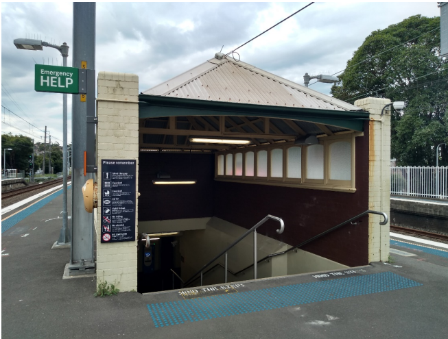
Figure 5.36: Entrance to stairwell lantern structure from Platform 2/3, facing north (Source: Jacobs 2020)
