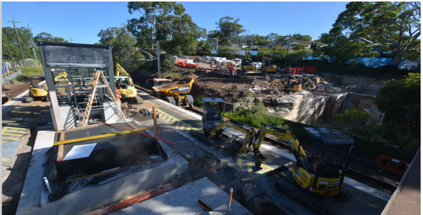
Image: Current progress on the station Platform under construction, February 2021
