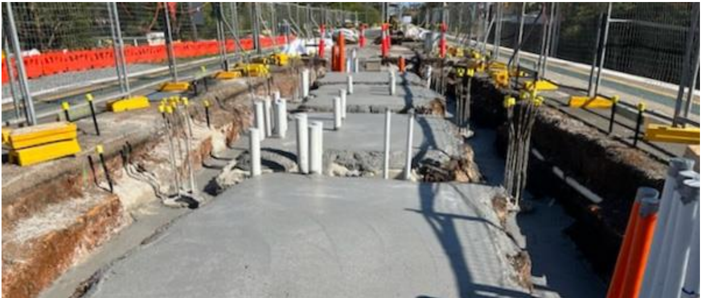
New building foundation with electrical and communications conduits.
