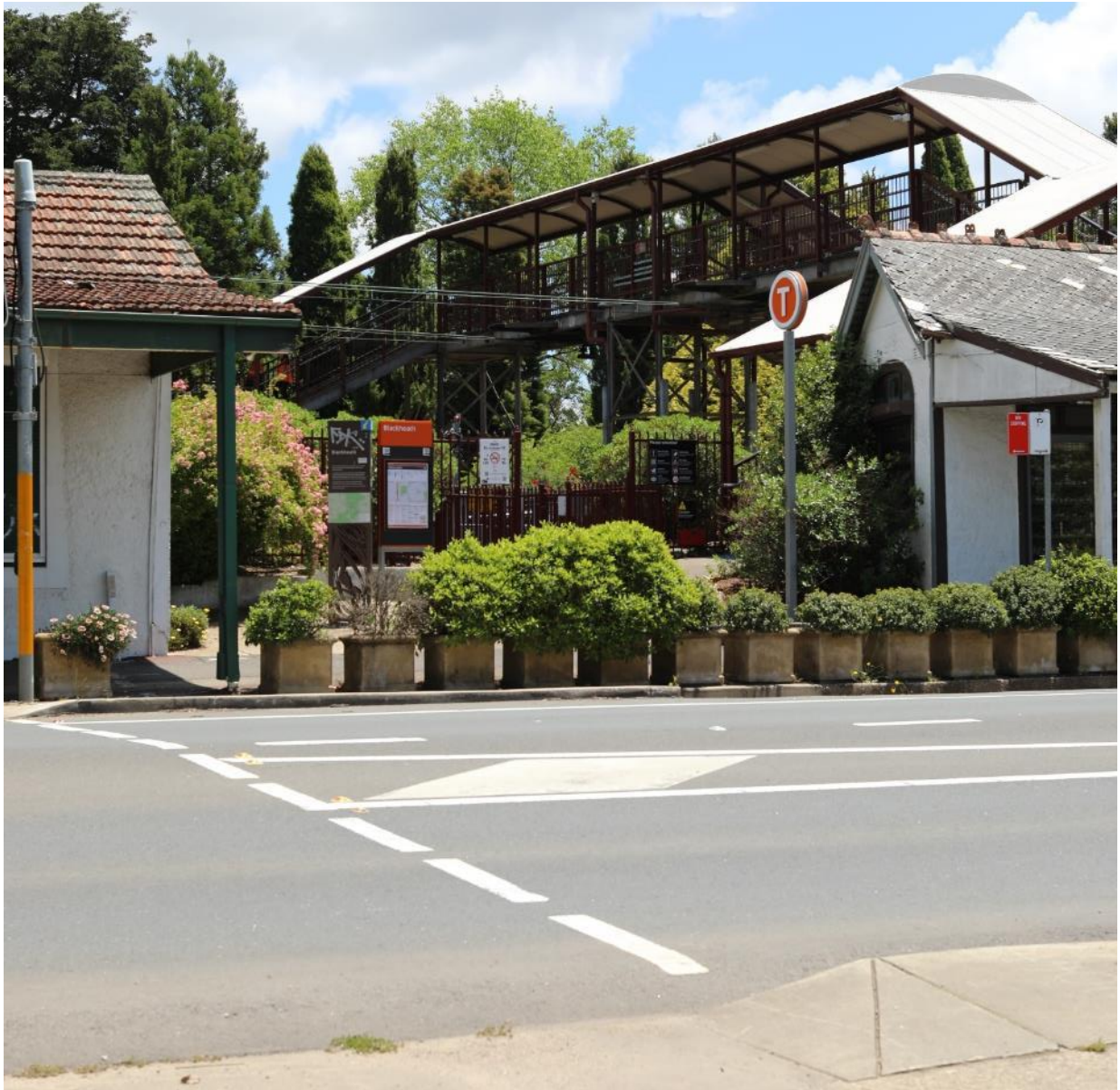
Photo 1.3 Station entrance from the Great Western Highway showing the pedestrian crossing and stairs, viewed eastwards towards Blackheath Station
