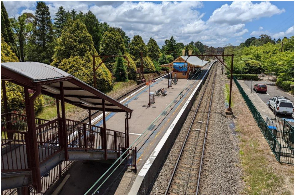
Photo 1.1 Station building, stairs and island platform, looking north from the footbridge
