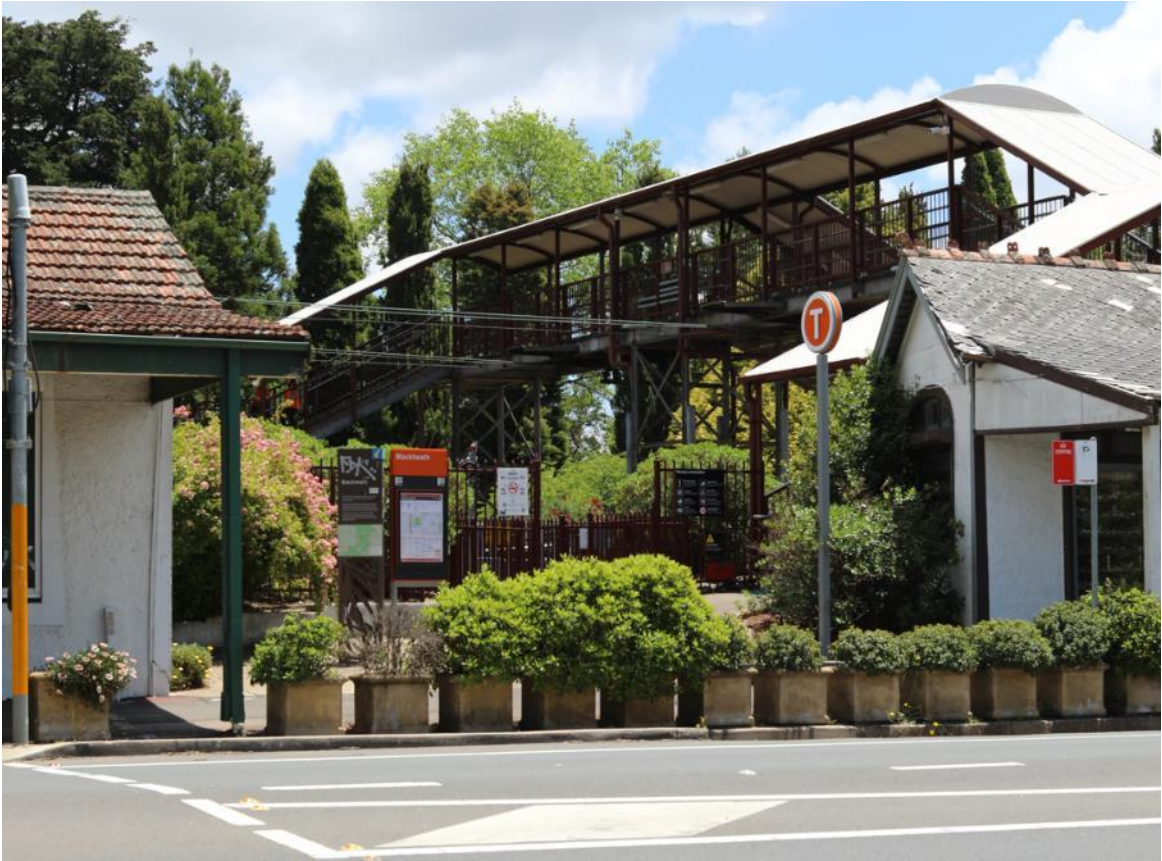
Photo 6.1 Access from the Great Western Highway
