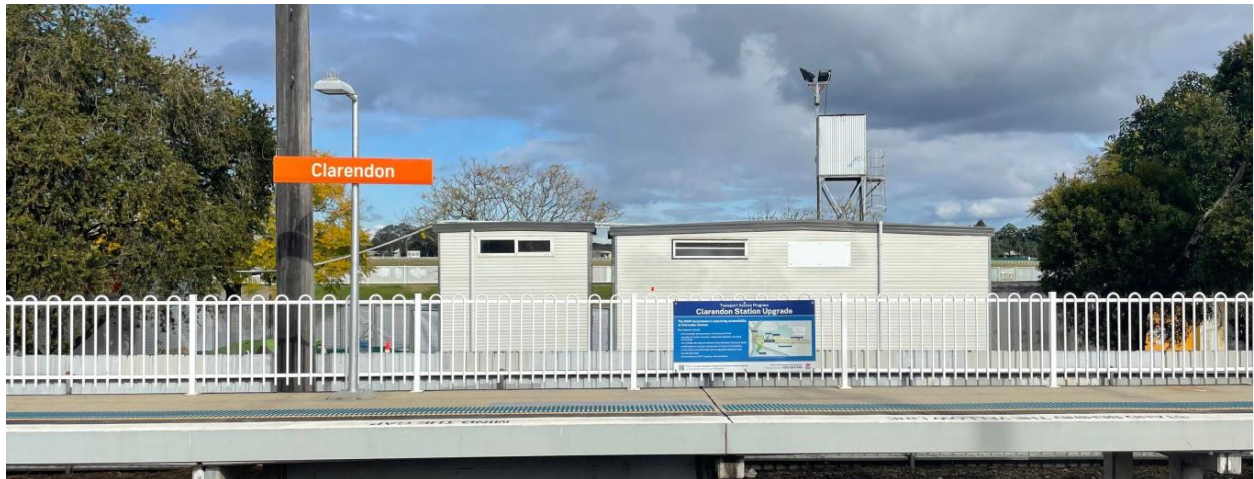
Clarendon Station Upgrade site sheds
