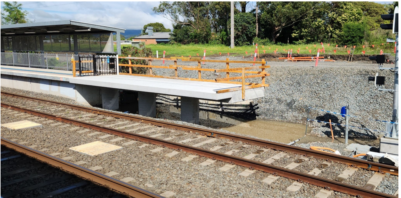
Platform extension work has been carried out at Dapto Station in 2022.
