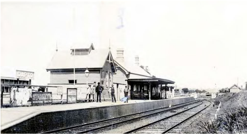
Plate 3.7 Dapto Railway Station, nd. Source: TfNSW 2022
