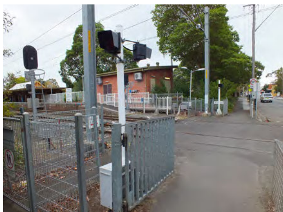
Figure 4.1 View from Bong Bong Rd level crossing towards entrance to Platform 2.
