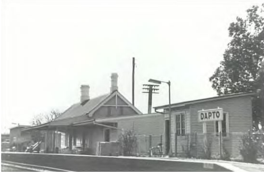
Plate 3.6 Dapto Railway Station, nd. Source: TfNSW 2022
