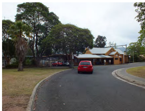
Figure 4.4 Circular driveway entrance to the main platform building on Platform 2; view from Station Street.
