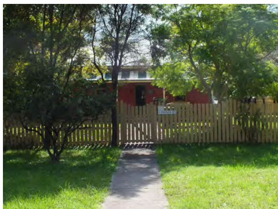
Figure 4.33 Path leading from the circular drive to former Station Master’s Residence (2012).
