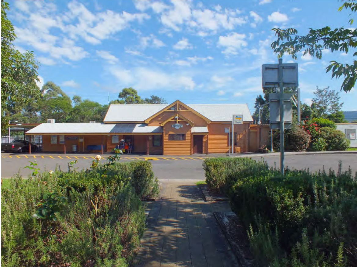
Figure 4.9 Original 1887 platform building on Platform 2; view from Hartigan Park (2012).
