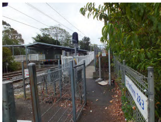
Figure 4.2. Ramp access to Platform 2.
