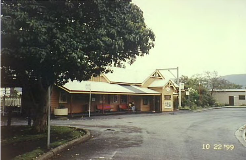
Plate 3.13 Dapto Railway Station 1999. Source: TfNSW 2022
