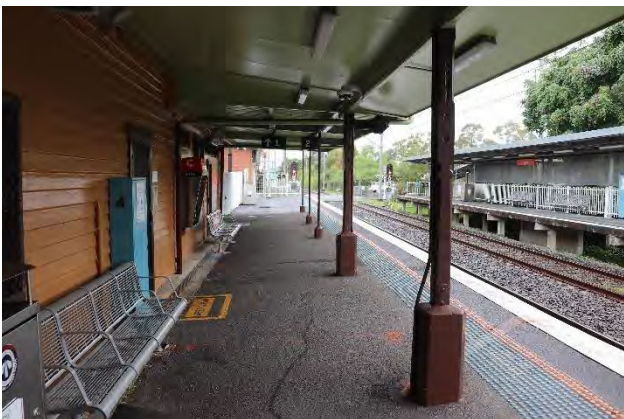
Plate 4.9 Platform 2 – southern end
