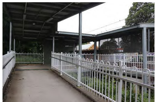
Plate 4.16 Ramp from level crossing at Bong Bong Road Platform
