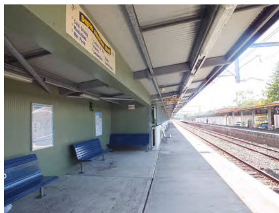
Figure 4.8 Interior of waiting shed on Platform 1 (2012).
