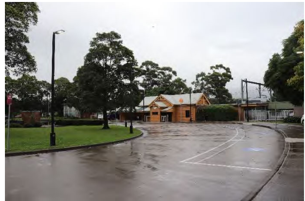
Plate 4.2 Dapto Station circular driveway
