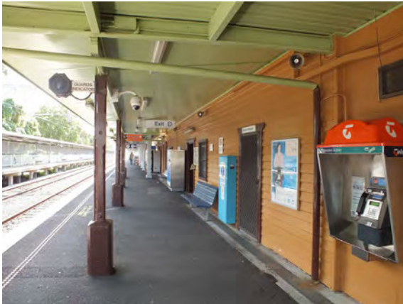
Figure 4.10 Awning supported by timber posts on Platform 2 (2012).
