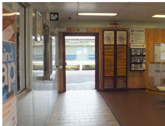
Figure 4.13 New ticket windows in the central waiting room of the main platform building.
