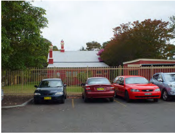
Figure 4.35 Rear of Station Master's Residence, separated from the commuter car park by a palisade fence.
