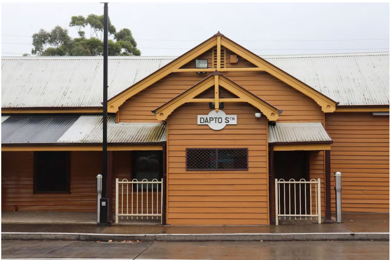
Plate 4.22 Awnings to Station Street elevation – central gabled station entry with flanking verandahs
