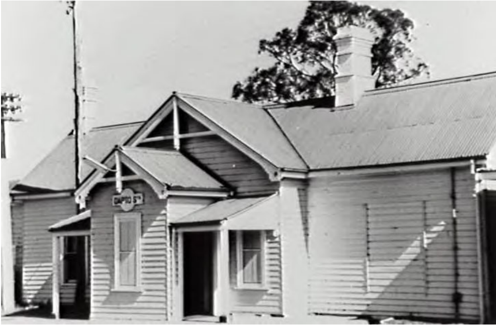
Plate 3.11 Dapto Railway Station 1981. Source: TfNSW 2022
