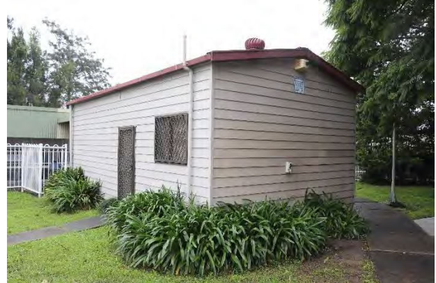
Plate 4.12 Weatherboard building to east of Platform 2
