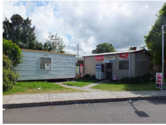
Figure 4.17 Demountable and shop building, north of the main platform building (2012).
