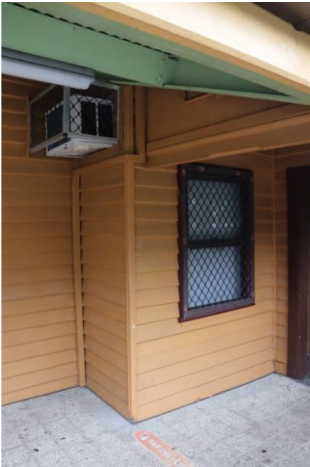
Plate 4.24 (left) Former southern verandah awning
