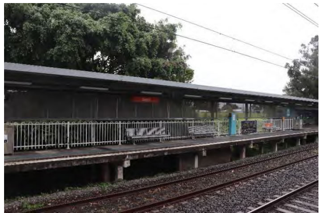
Plate 4.10 Platform 2 – northern end – precast post and beam structure
