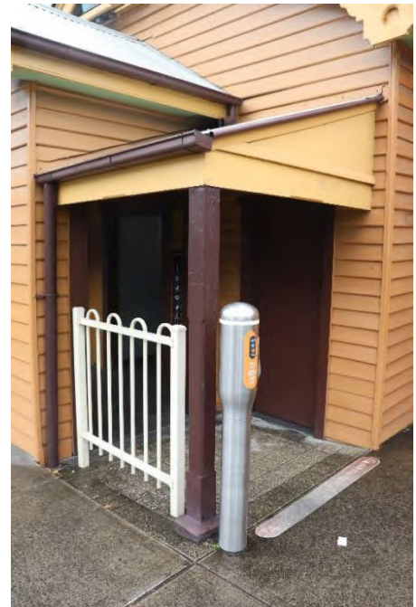
Plate 4.25 (right) Northern verandah awning have early fabric including timber side cladding and beams
