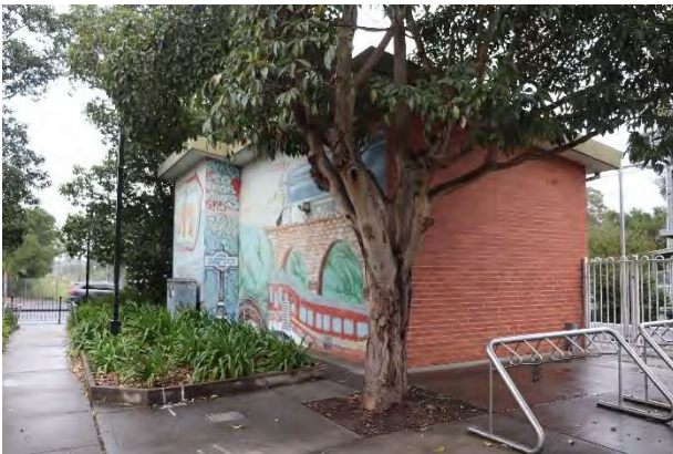
Plate 4.13 Brick signal relay room along Platform 2
