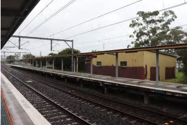
Plate 4.11 Platform 2 northern end combined with Platform 3
