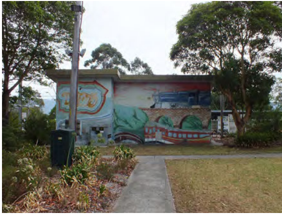
Figure 4.16 Brick relay room with painted mural at the south end of Platform 2.
