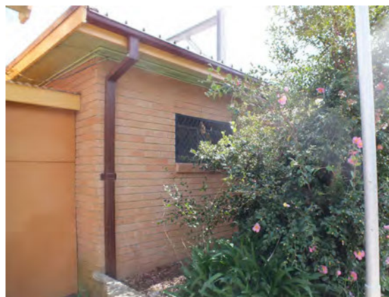
Figure 4.15 Modern toilet block, attached to the north end of the main platform building (2012).
