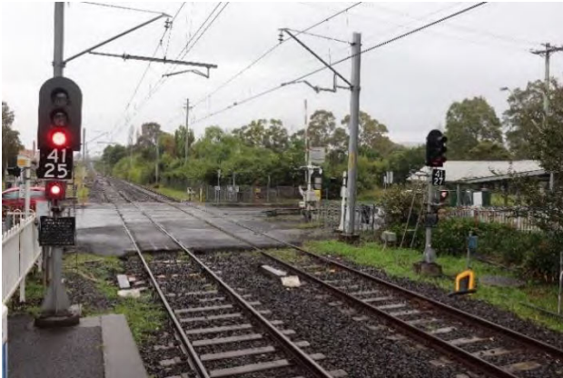
Plate 4.17 Level crossing at Bong Bong Road
