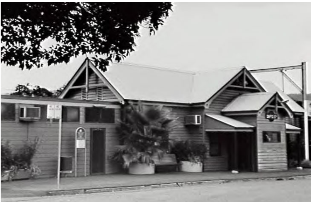
Plate 3.12 Dapto Railway Station 1994. Source: TfNSW 2022
