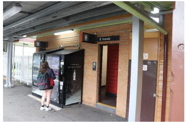
Plate 4.14 Pale brick toilet block along Platform 2
