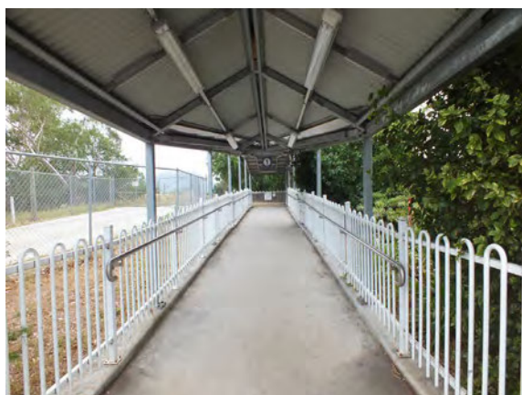
Figure 4.3 Ramp access to Platform 1.
