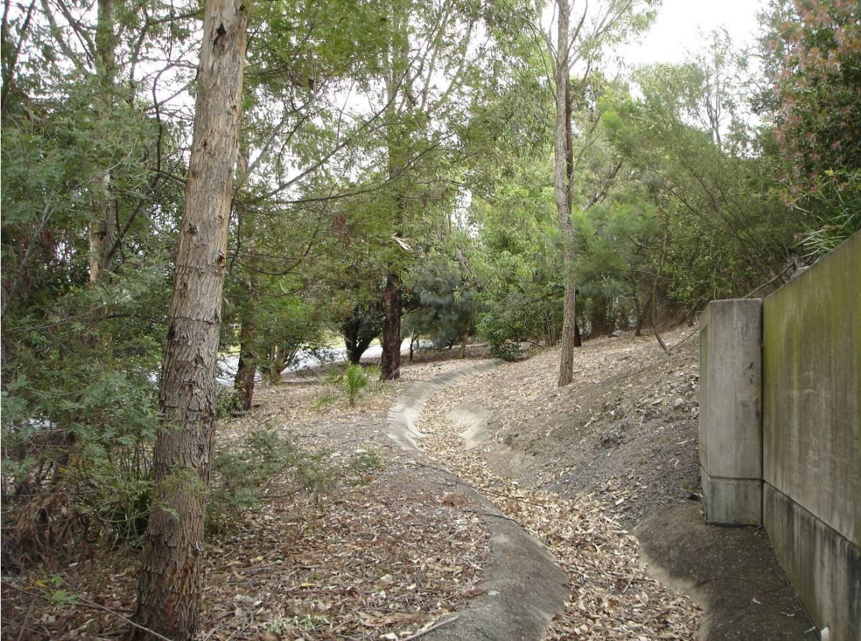
Photo 1 Concrete drainage channel and vegetation at Junction Road
