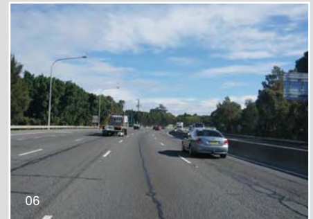
04 M4 - section of elevated viaduct between xxxx Photography by HASSELL
