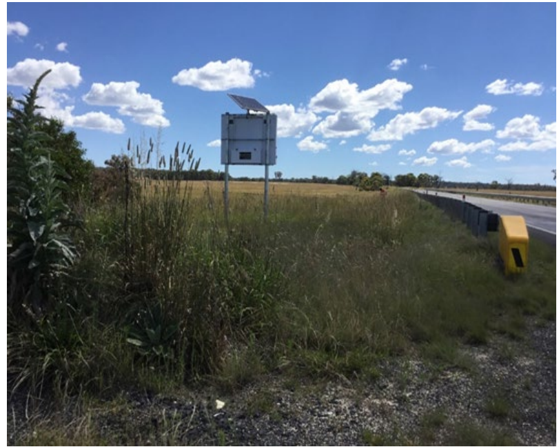
Plate 3-6: PCT 567 (low condition) in study area
