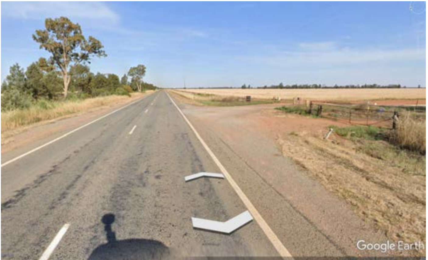
Figure 6-2 Typical private property access along Burley Griffin Way (Source: Google Earth)
