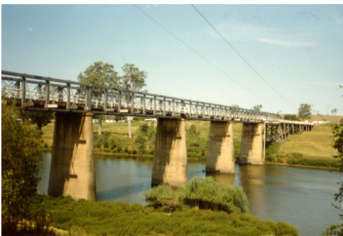
Solutions beyond the limits of timber beam bridges, left, timber trusses on concrete piers over the Clarence River at Tabulam, right, iron lattice trusses on cylindrical iron piers over the Snowy River at Dalgetty.
