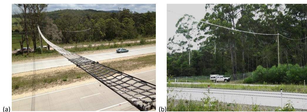
Plate 1: The rope bridge at Kew features two spans – one over the dual carriageway and a second over a service road to the west (a). The single-span John's River rope bridge connects directly to forest on the west (b) and east sides of the highway.
