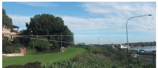
This carefully scaled and well sculpted and landscaped noise mound adjacent to the City West Link in Sydney not only blocks noise from traffic but allows views of the harbour.
