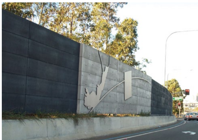
City West Link: A successful urban design outcome achieved through collaboration between engineers, urban designers and artists.
