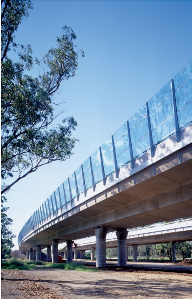
Angled clear noise walls with tapered supports, integrated with the road viaduct, where the whole is considered as a three-dimensional composition as on this M7 Motorway viaduct.
