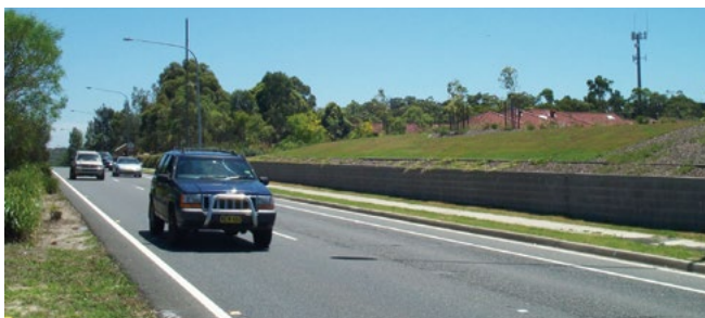
A noise mound is a better urban design solution for road users and residents than a noise wall in most instances.
