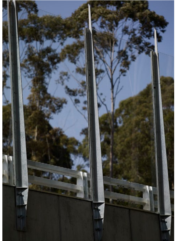
Transparent acrylic panels used on Bonville Bypass on the Pacific Highway allow views from bridges of the landscape.
