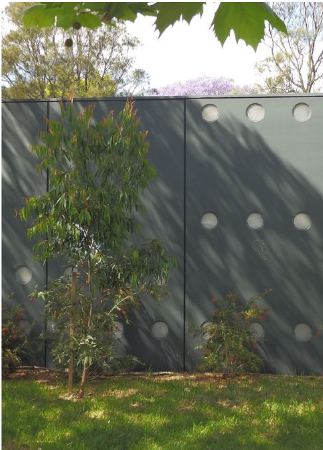
The walls on Syd Einfeld Drive are designed to protect the park and streets on the residential side and provide a human scale. They have a dark grey recessive colouration. There is great attention given to proportion and articulation of panels and to detail, such as the acrylic portholes.
