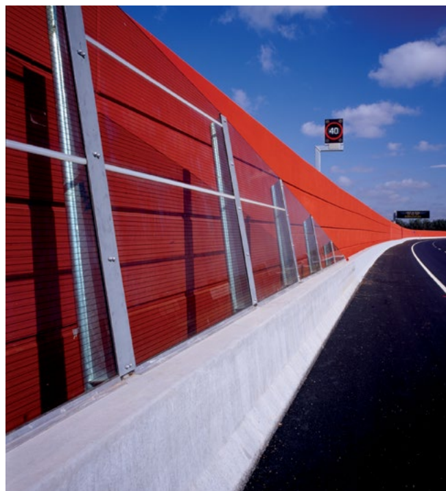
Noise walls provide road users with a visual experience in movement.
