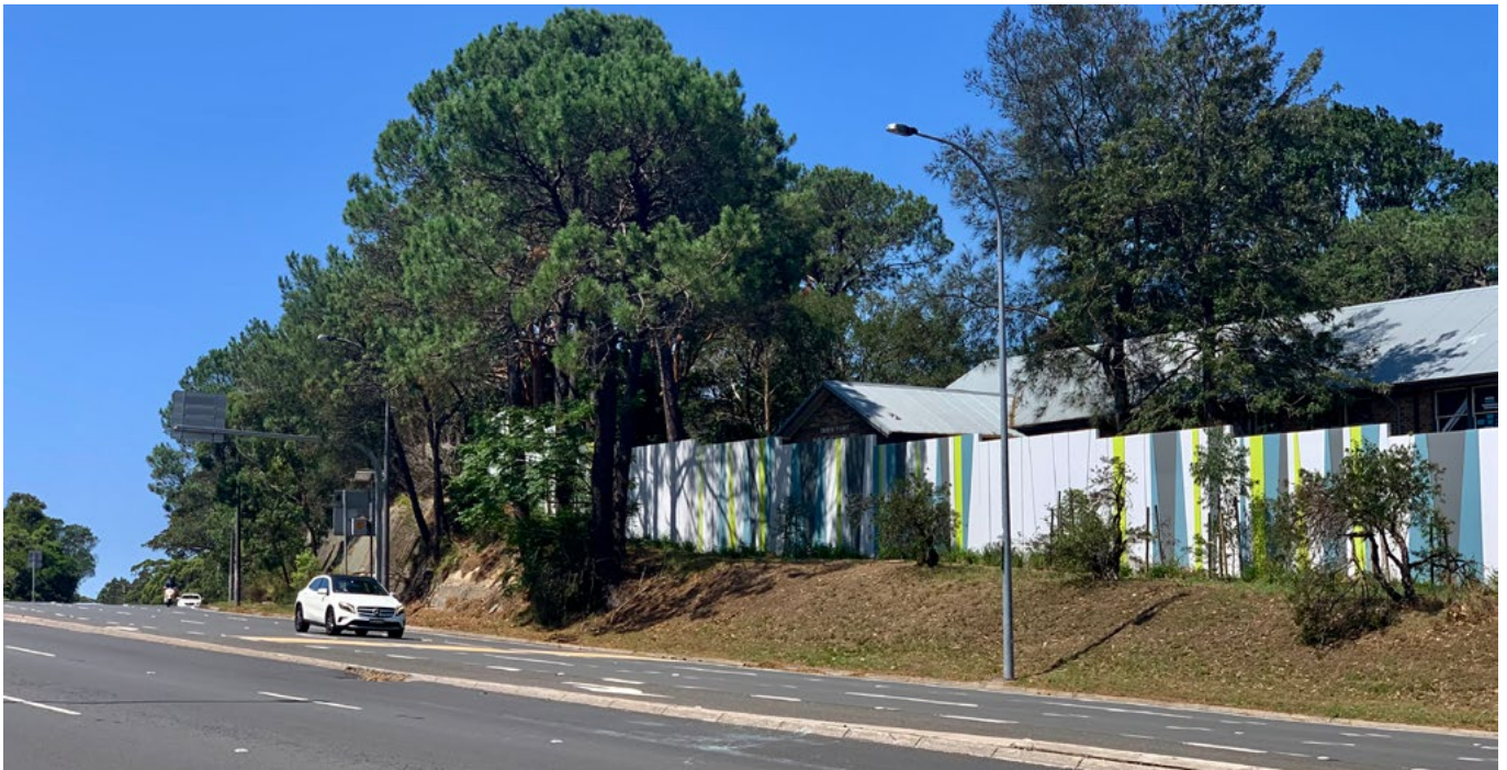
A short noise wall protecting a primary school on Taren Point Road. Concrete walls with playful colouring and patterns to reflect the school and its pine trees. Small regular steps work well to accommodate the slope and importantly retaining existing trees outside the wall helps set it into the landscape.
