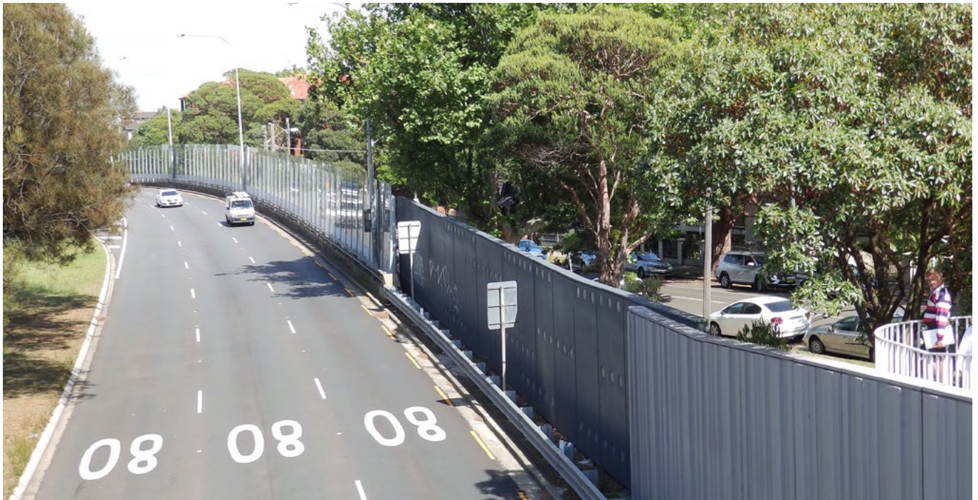
Syd Einfield Drive: A composition of noise wall types designed to address different conditions on the road and residential side but unified and context sensitive.
