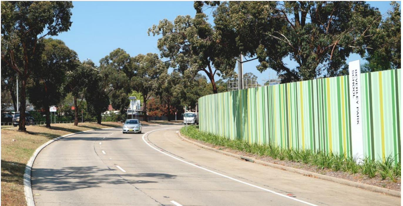
A system of interlocked concrete noise walls protects two Campbelltown schools at Thomas and Moore Streets and helps define this precinct.
