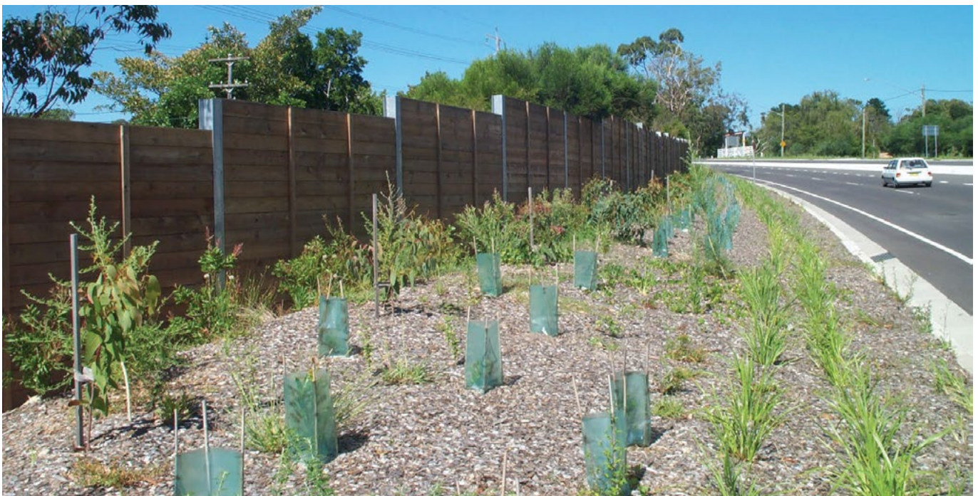
Timber has a domestic scale, and needs to be well articulated in its context.
