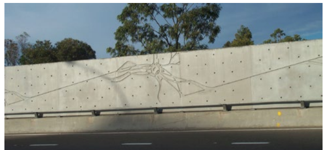
Strong noise wall patterns on a section of the M4 Motorway.
