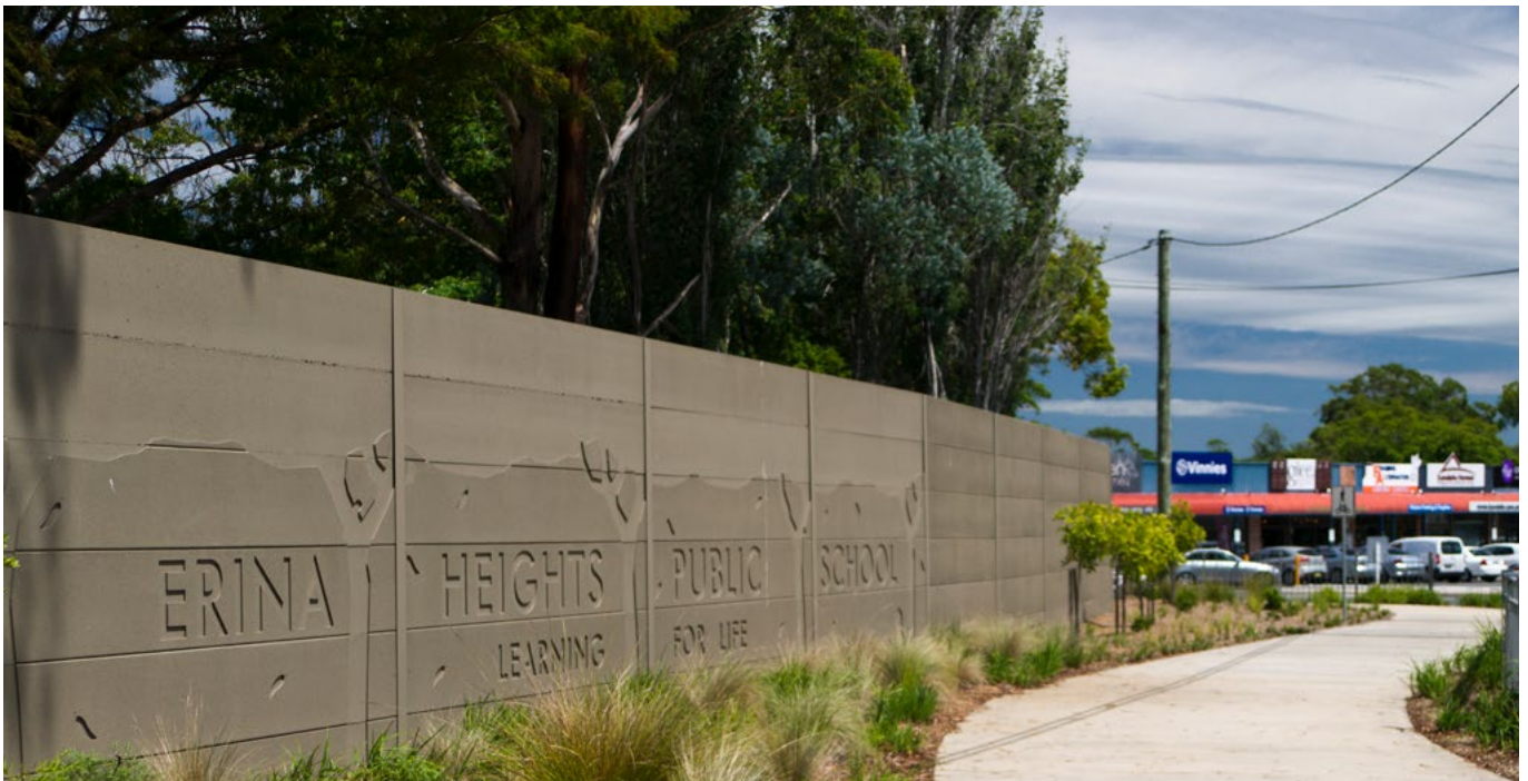
This neatly designed wall with lettering protects Erina Heights Public School from noise and fronts onto landscaped public space with shared path.
