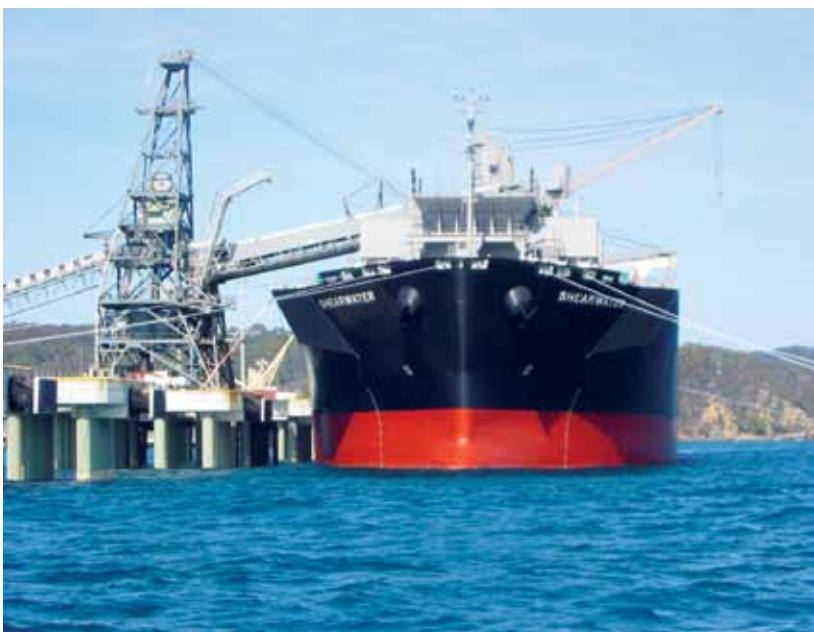
A ship berthed at the multipurpose wharf in Eden.
