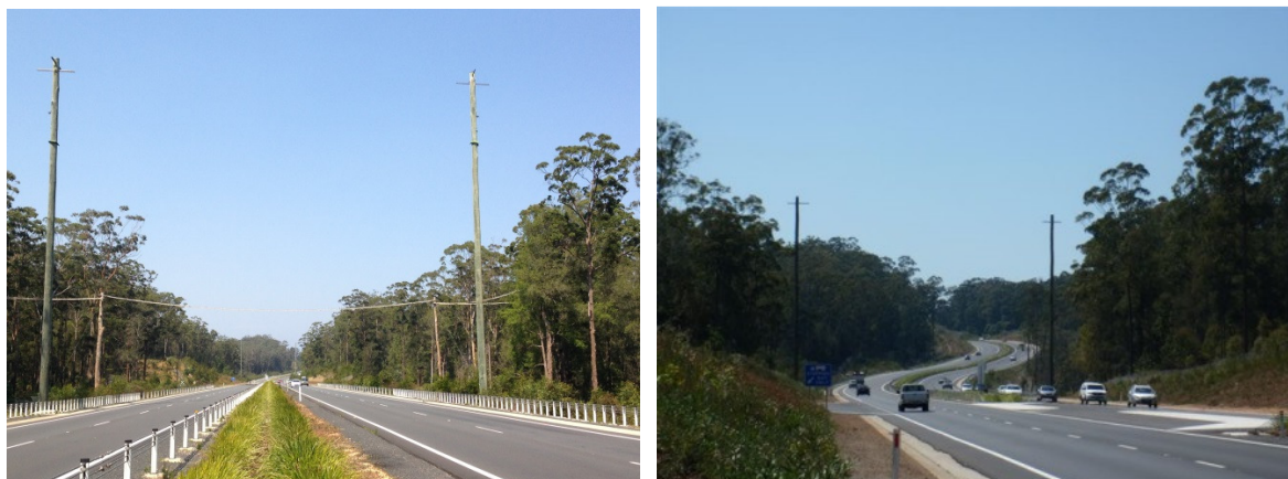
Figure 2. Glide poles on the Oxley Highway. At left the western pole pair and at right the eastern pole pair.
