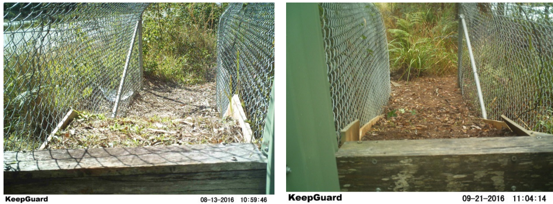
Figure 10. View looking down a drop-down ramp into the road-side vegetation for drop-downs 5S (left) and 7N (right). This shows the substantial amount of road-side vegetation that may be attractive to animals for foraging.
