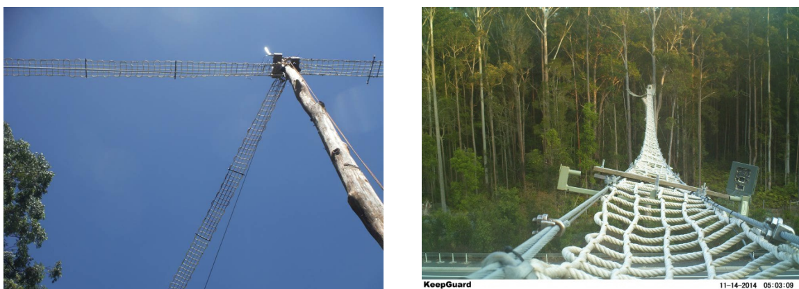
Figure 6. Attachment of the rope-bridge to a supporting pole. There are two sections of the rope-bridge that allow access from trees in the forest ( Left ). Photograph taken at the south end of the rope-bridge. The Reconyx camera can be seen to the right of the rope-bridge ( Right ).
