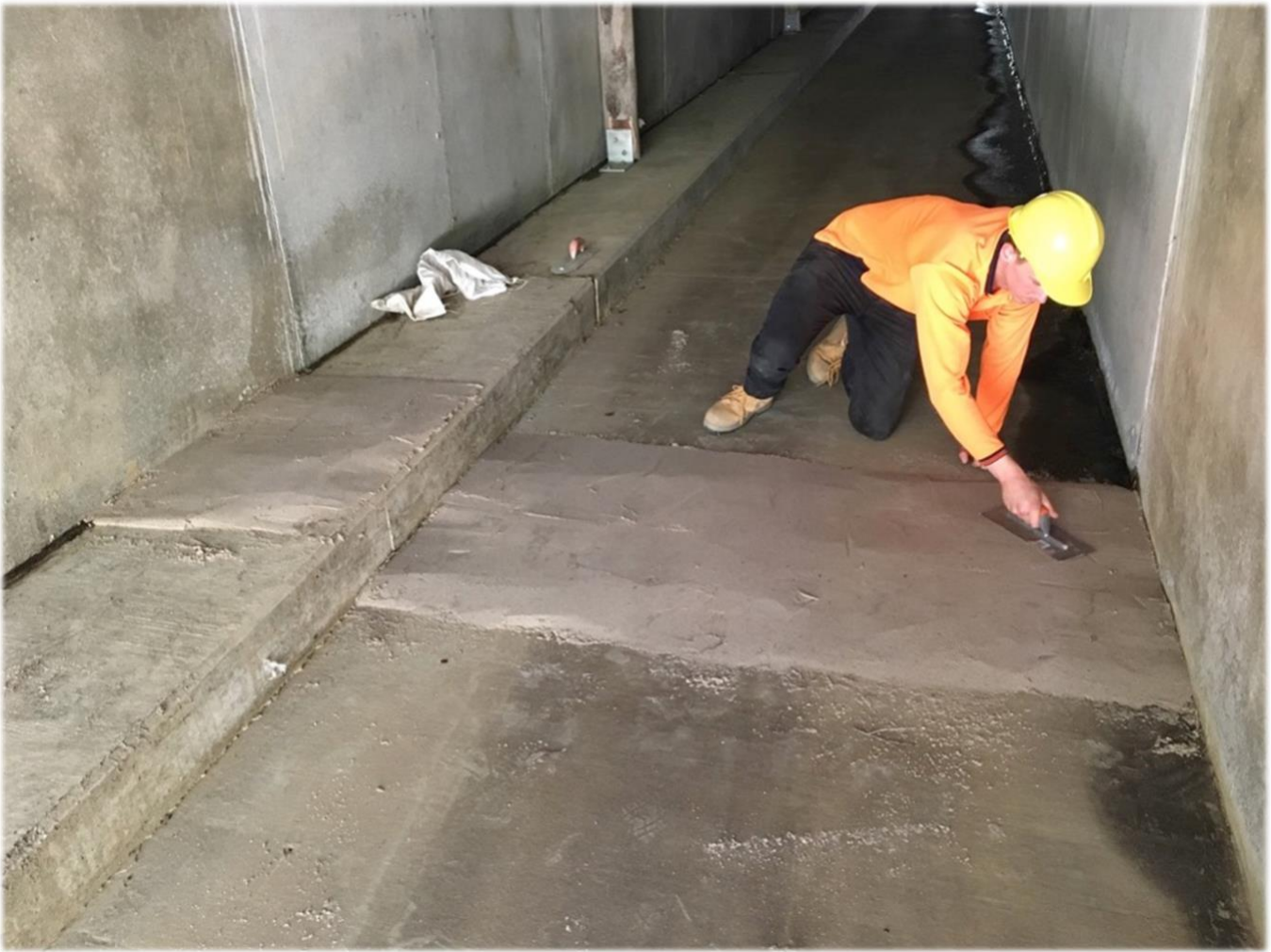
Plate 2: Sand pad being installed in a fauna underpass on the WC2NH upgrade.
