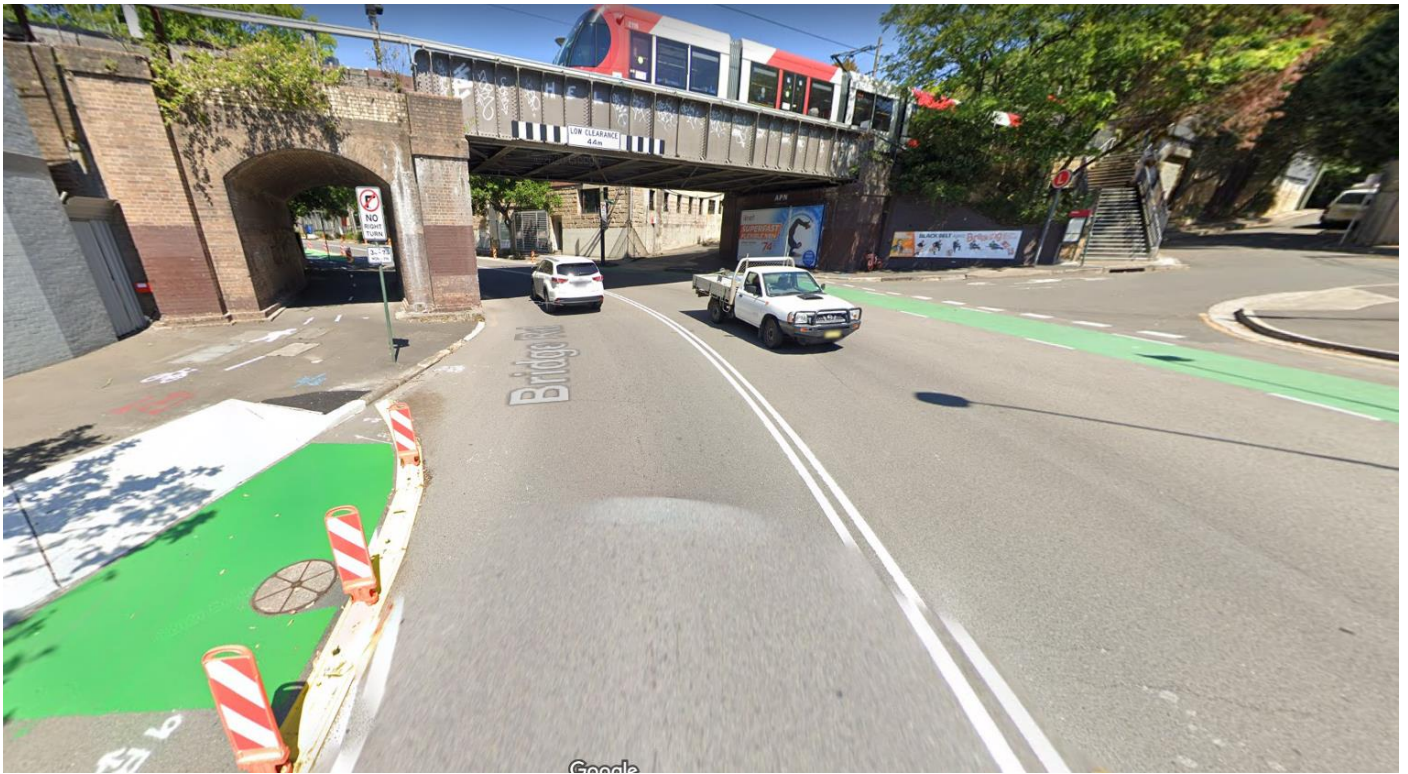
Figure 6-2 Viewpoint 1 Bridge Road near Burton Street looking south near tram overpass
