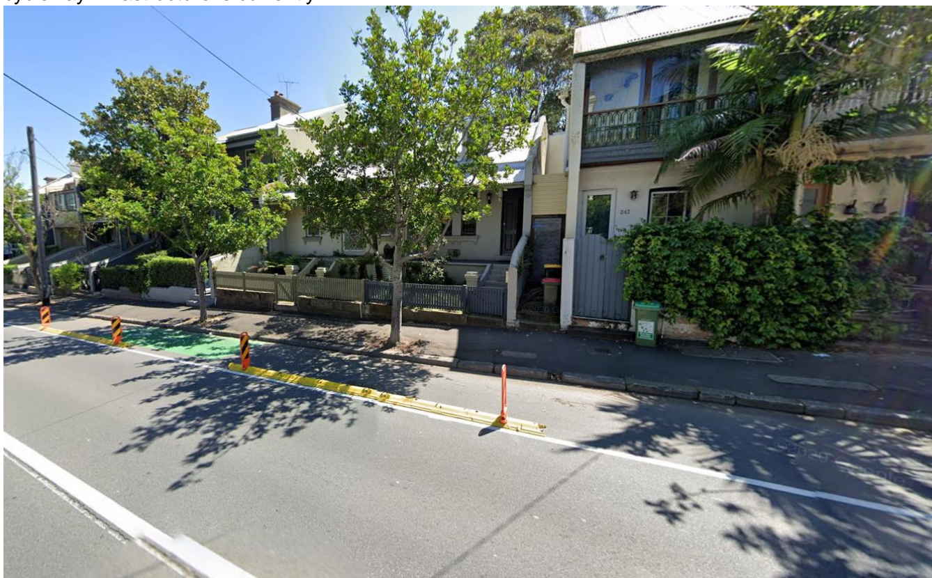
Figure 6-7 Viewpoint 6 Bridge Road opposite Junction Street
